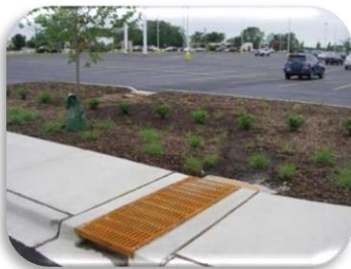
Parking lot retrofits in St. Charles, IL
