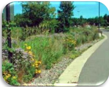
Curbless street with infiltration strip in MN
