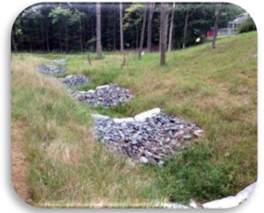
Regenerative stormwater conveyance system in Baltimore County, MD
