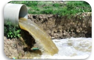
Stormwater outfall in Baltimore County, MD
