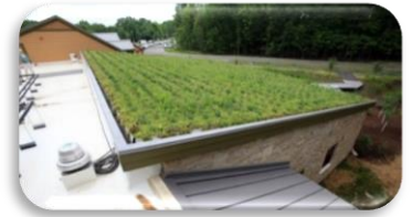
Green roof at West Creek Reservation's Watershed Stewardship Center in Parma, OH
