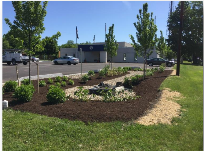
Bioretention cells retrofit in Madison Township, OH
