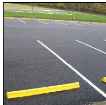
Porous asphalt within a parking lot. Credit: Chagrin River Watershed Partners, Inc.
