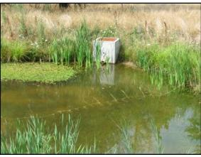
Outlet structure with multiple drains **free of obstruction** such as vegetation, trash or sediment.
